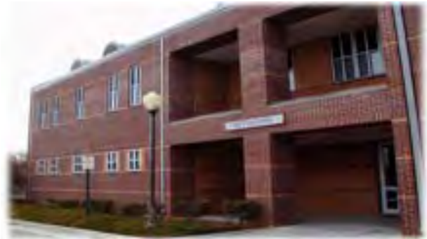
Roswell Police Department Detention Center
